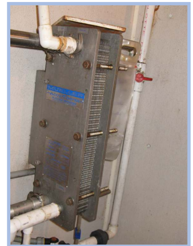
Heat exchanger for well water precooling of milk. Photo courtesy of Penn State Extension.
