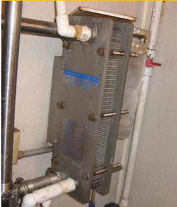
*This heat exchanger at a dairy farm precools milk using well water. It's just one of many energy efficient measures an assessor might recommend. (Photo courtesy of Penn State Extension.)*
