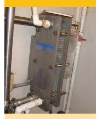
This heat exchanger at a dairy farm precools milk using well water. It's just one of many energy efficient measures an assessor might recommend. (Photo courtesy of Penn State Extension.)
