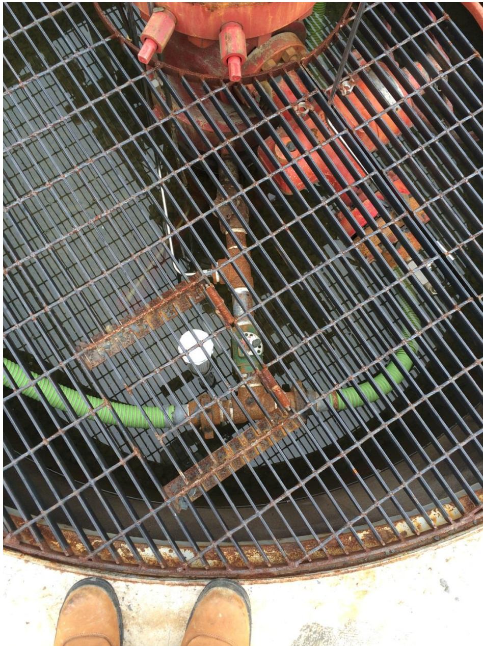
IMAGE 2. Photograph showing green flexible line that can be heard gurgling and seen visibly surging. Observation may indicate transfer of fluid to the annuli of other wells. It appears that operator does have a way to isolate the annuli; however, one well may be adding gas to the annulus of another well that is not making any gas. Wells with annular gas are difficult to verify unless each well is isolated and allowed to vent for a time period to establish a baseline condition from which an accurate observation can be made. This well configuration could result in DEP believing that gas is present outside more annuli than is actually the case.
